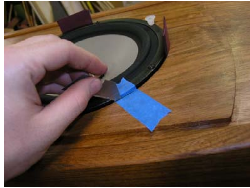
Cut the tape in order to remove the driver and deepen the holes to the proper depth.
