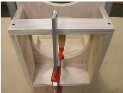
Front side bottom shown with all pieces installed
